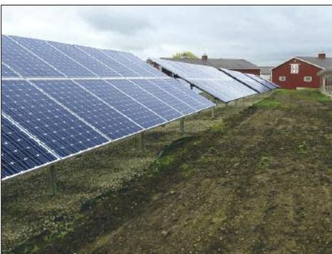
six electricians based out of IBEW Local 103 throughout the project. The system is comprised of 760 solar panels mounted to a ground-mount racking system, covering about an acre of Mann Orchards 29-acre site. The panels are intercon-
