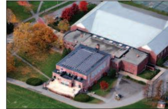
Adam Palmer and Foreman Paul Kelly. The system consists of 154 Kyocera solar panels and two (2) Solectria 15kW solar inverters, and a PanelClaw ballasted roof-mount system. ■
