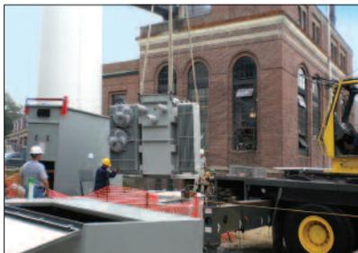
Padmount transformer being offloaded for installation at UNH heating plant facility. It steps up supplemental generator voltage from 5kV to 38kV and interconnects to the Public Service power line.
