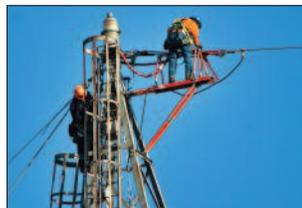
harnesses. A helicopter was also utilized to allow for disengaging four (4) aviation obstruction safety balls from the existing cable line, enabling line inspection. The procedure was necessary to ensure the integrity of the existing line was
