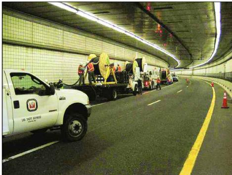
*The NECA contractors' project scope included the installation of more than 13 miles (70,000 feet) of 4 runs of 72 strand fiber optic cabling and 12,000 feet of coaxial cabling*
