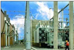
The electrical project scope for the facility includes construction of an enclosed 345kV/115kV Mitsubishi Gas Insulated Substation (GIS) with four (4) 448 MVA auto-transformers. Within its scope of work, State Electric provided installation of a completely redundant control and protection system, housed within a multi-room control building. The GIS equipment is contained
